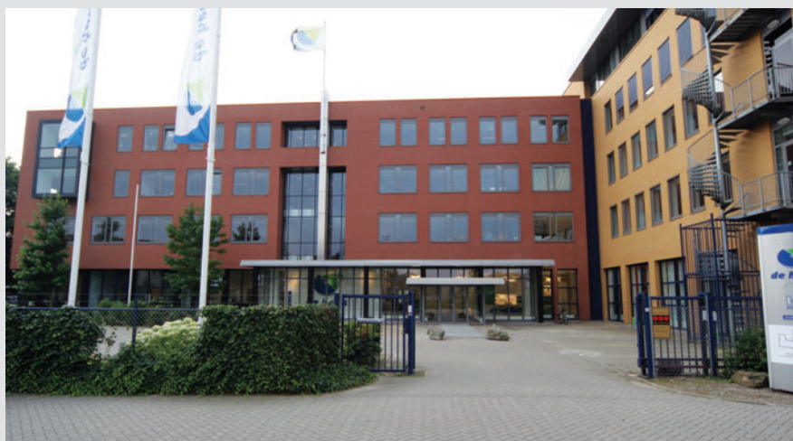
The new plant has a capacity of 120,000 tonnes. (Photo: De Heus)
